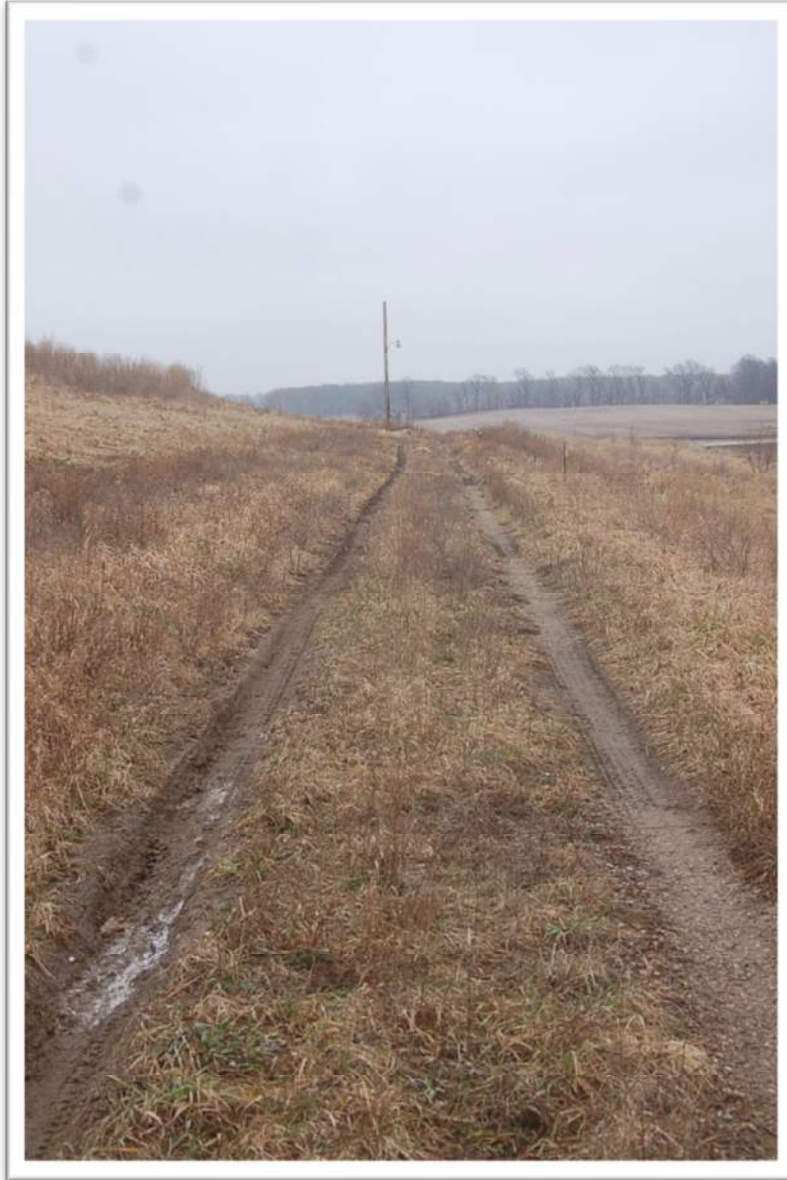
6. Mid section of South Slope Facing West Middle of Slope
