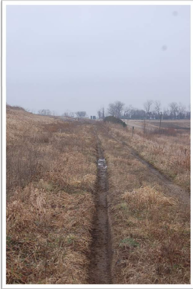
2. West End of South Slope Facing East Middle of Slope
