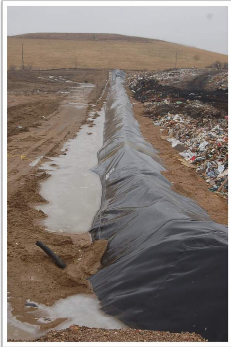
17. Near Middle of Site Facing East Lined Outer Berm
