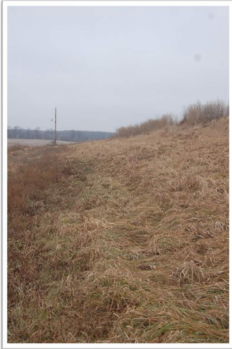
4. Mid section of South Slope Facing West Top of Slope
