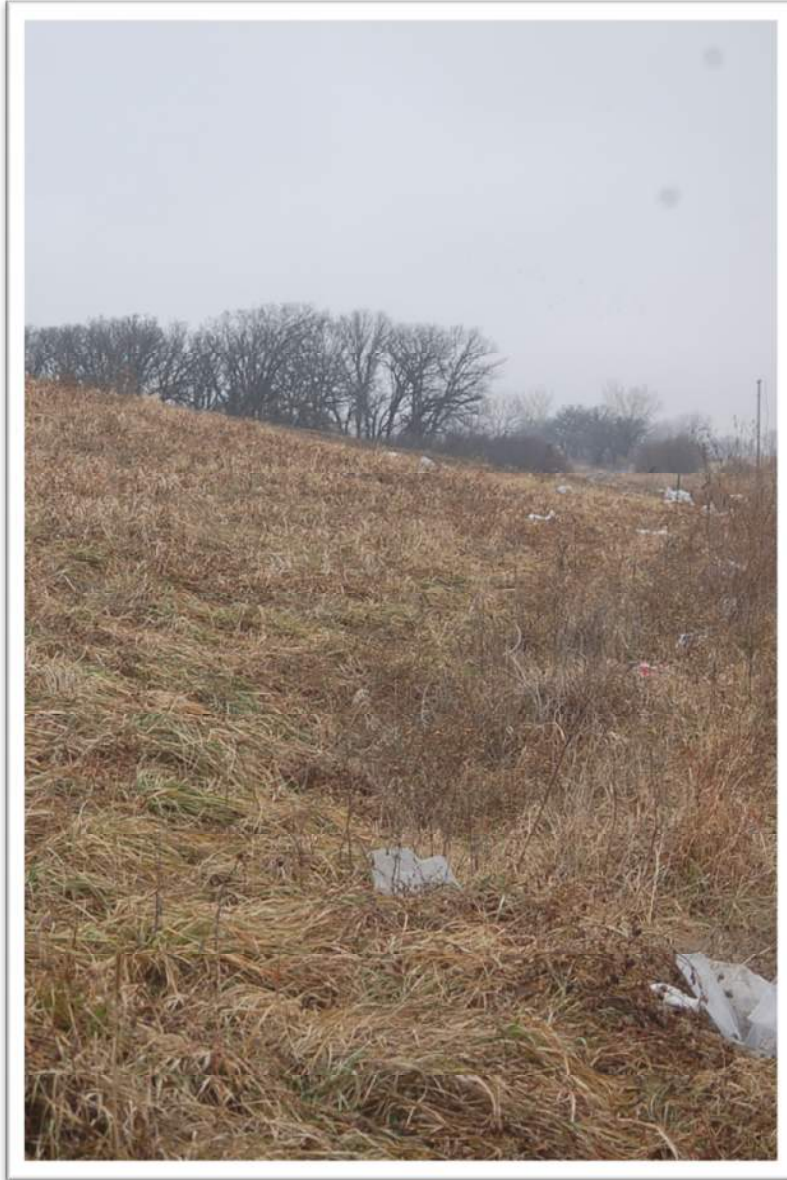
12. South End of East Slope Facing North Top of Slope
