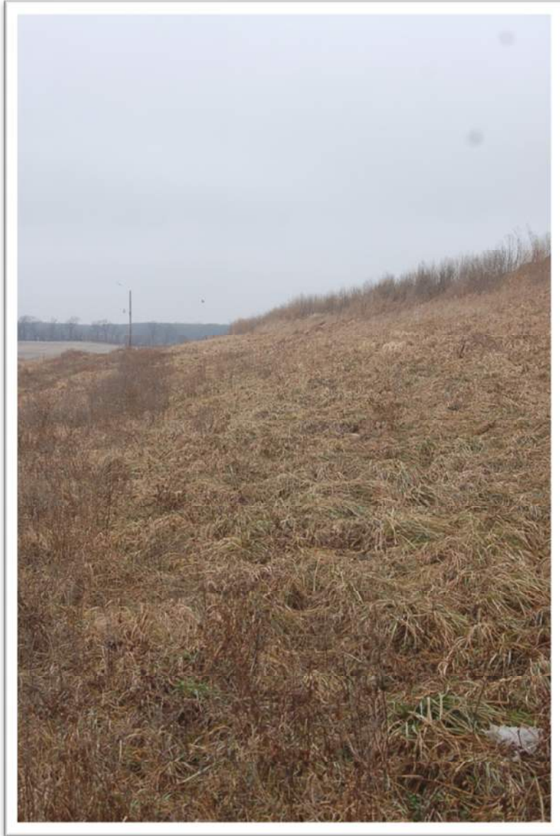
10. East End of South Slope Facing West Top of Slope
