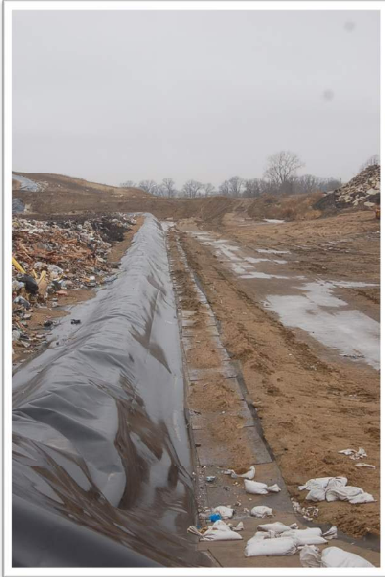
16. East Side of Site Facing West Lined Outer Berm
